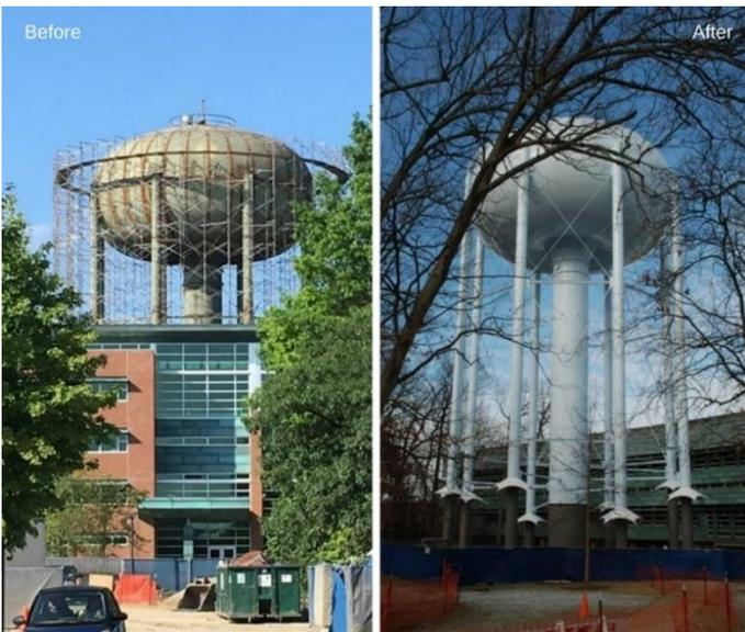
Caldwell Tanks tore down the existing tank, and then fabricated and erected the new tank pictured on the right. CCC painted the tank as a subcontractor to Caldwell Tanks. Now, the project just needs a new fill pipe to be completed! In the project photos below, you can see just how tight the construction site was that the contractors and painters dealt with.
