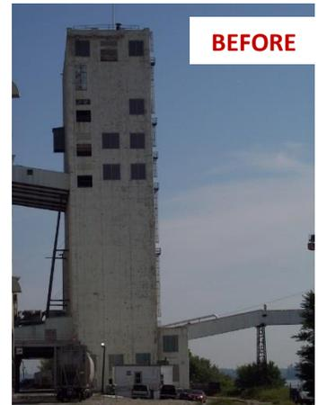
Needless to say, the chosen product needed to be a true “dry-fall.” The new paint had to have great adhesion to both previously-coated (read old paint) and uncoated concrete *and* metal. The new coating had to have mold and mildew resistance *and* be available in a low sheen finish. Consequently, it didn’t take long to recommend Induron **Aquanaut II Low Luster**.
